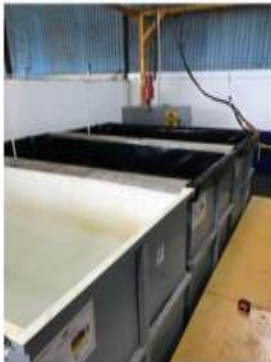
Alkaline Cleaning Line 3 Tanks
