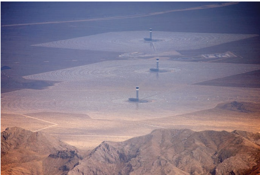
Fig. 7.11 Ivanpah solar power plant, creative commons license-photo by Craig Butz
