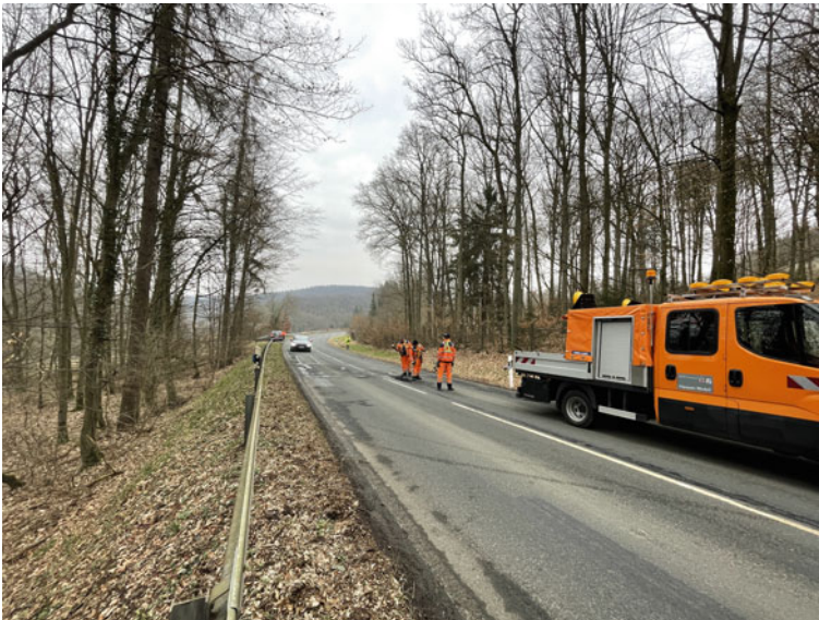
Fig. 1 Short-term roadworks site
